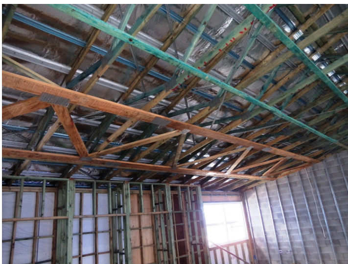
Example of a Wind Truss Installation
